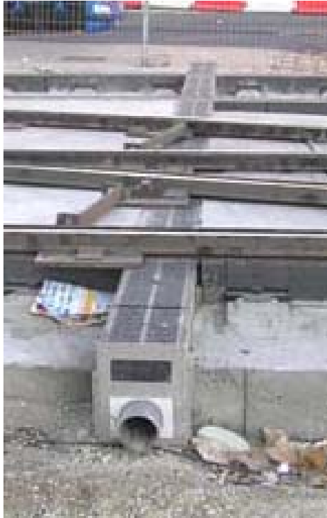
Transverse drain in Montpellier E Hollis
