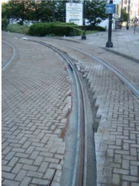
Rail concreted in place
