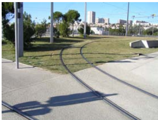
Street and segregated track in Montpellier
