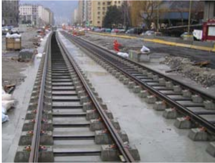
Twinblock concrete sleepers for street track in Grenoble E Hollis
