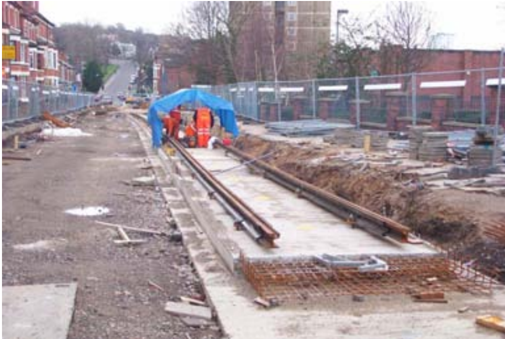
Pre-coated rail installed on concrete slab
