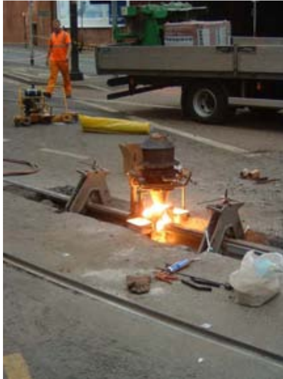
Welding a rail joint
